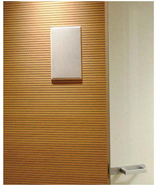
UN ALTRO PARTICOLARE DELLA SALA HOME THEATER: IL DIFFUSORE SURROUND DESTRO, FISSATO SUL RIVESTIMENTO ACUSTICO DELLA PARETE. I DIFFUSORI SONO PILOTATI DA UN SINTOAMPLIFICATORE DENON AVR-X4000 DA 7 X 165 WATT (SU 6 OHM), CHE FORNISCE UNA POTENZA PIÙ CHE SUFFICIENTE A SONORIZZARE LA PICCOLA SALA.
